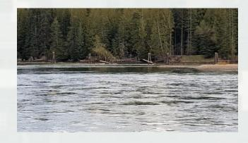
Wing and waves cause the boom to fail due to forces on aged and fatigued parts.
