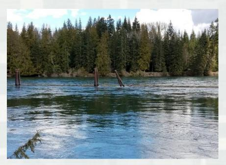
Dolphin Damage - Parts failing. Ex. One piling broke and the other two were twisted downstream. (note: This dolphin completely failed in 2017 and has been replaced)
